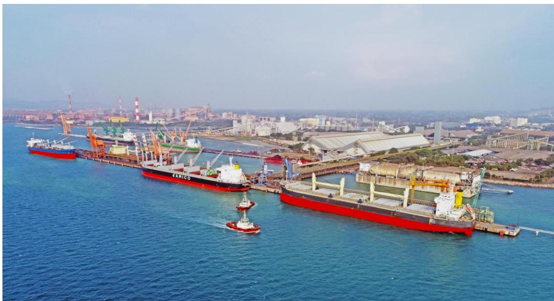
Port of PT Krakatau Bandar Samudera, Indonesia
